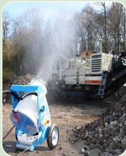
De-odourant guns during excavation
