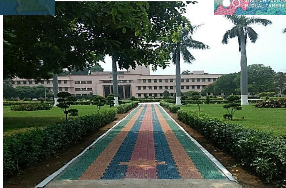
Waste Plastic tiles reinforced with fly ash installed at CSIR-National Physical Laboratory, New Delhi
